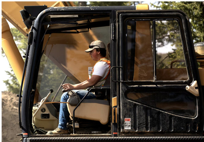
19-year-old Tristan Hoepfner loads blast rock into a truck at Hidden Trails.
